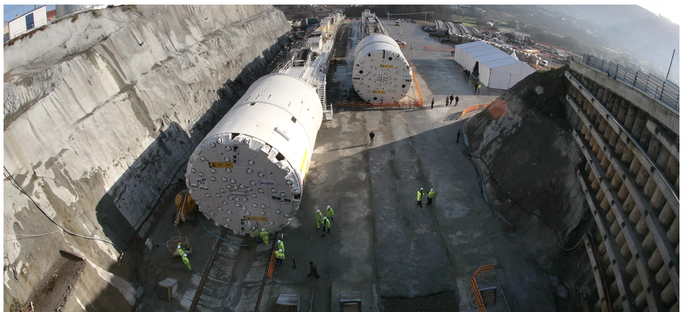
Boring the north Vigo access tunnels.
